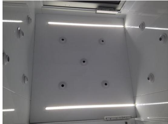
**Photo 32:** Typical Air Shower/Tunnel LED lighting
