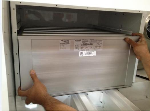
*Photo 30: HEPA filter shown being removed*
