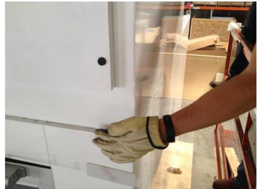
**Photo 16:** Blower Module shown manually pushed into place
