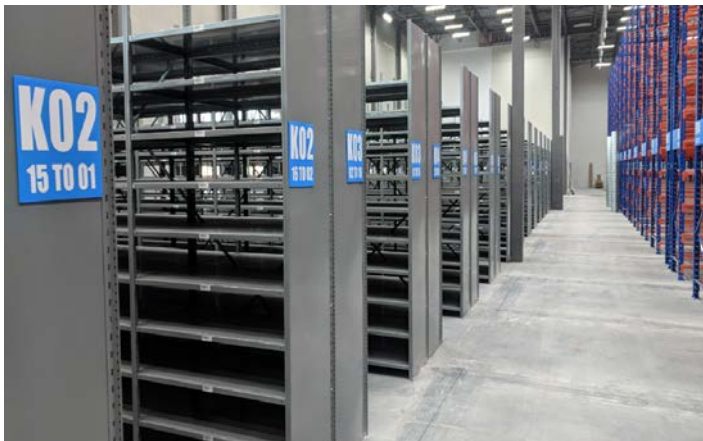
Interlok shelving in a distribution center for tools and hardware products.
